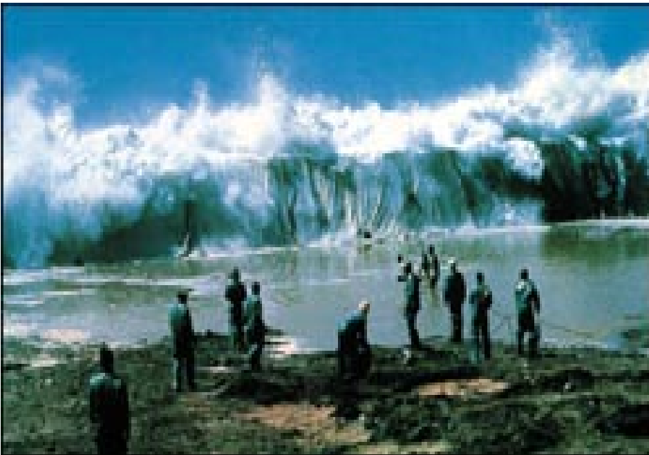
Above: Sea-walls give access to offshore diamond-bearing gravels
